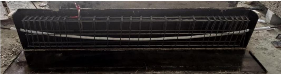
**Figure 2:** Reinforcement cages
