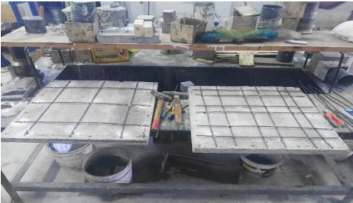
Fig. 16: Strengthening of slabs with steel bars
