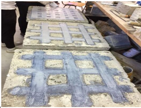
Fig. 17: Strengthening of slabs with fiber glass and carbon fiber sheets
