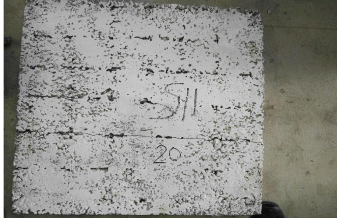
Fig. 19: Reference Slab (S11) with Reinforcement 7x6 mm in both Directions (Fcu =22 mpa Pu=23.32kn)
