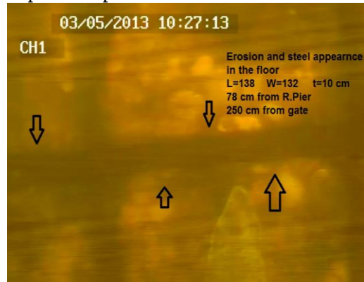
Photos (9) and (10): Floor Steel Erosion
