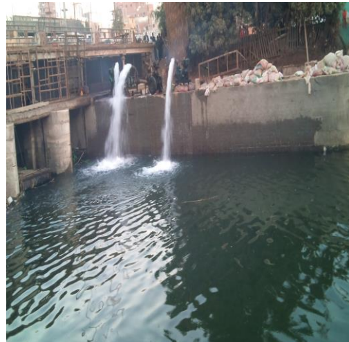
Photo (12): Pumping water out of the vent
