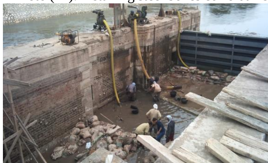
Photo (13): Cleaning the vent after water is pumped
