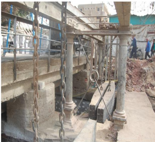
Photo (11): Installing steel boxes cofferdams
