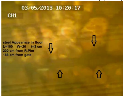
Photos (9) and (10): Floor Steel Erosion
