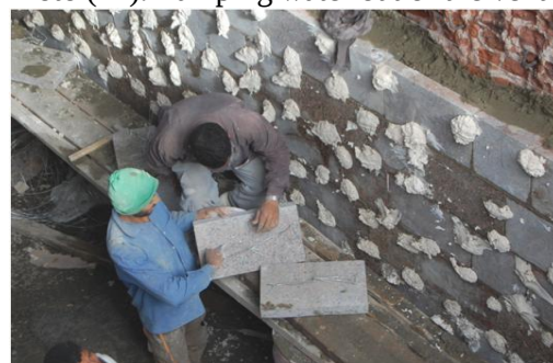
Photo (14): Vent Repair
