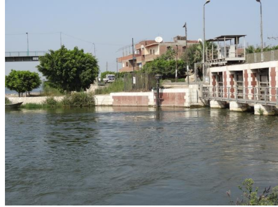
Photo (4): Wing wall, D.S.
