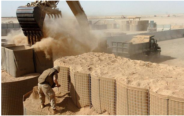
Fig. 4: Installation of Hesco barrier [19]
