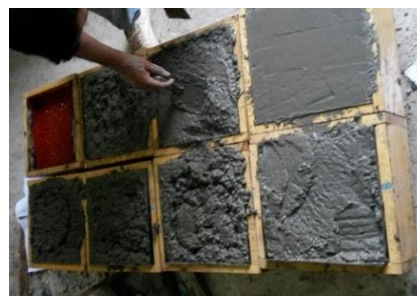
Figure (6): Finishing of overlay concrete
