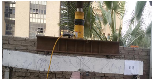
Fig.4 Mode of failure for group 1.
