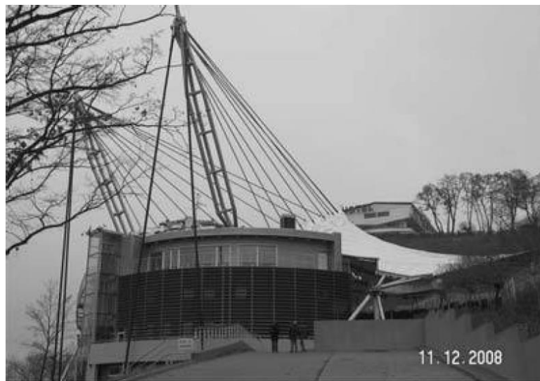
Figure 1. Roof and pylons of amphitheatre structure considered.
