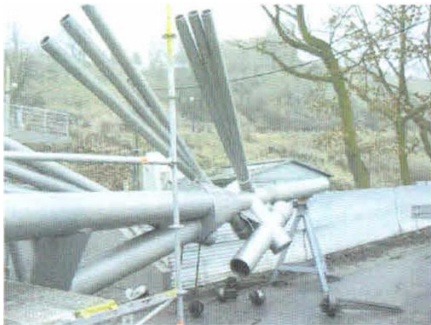
Figure 2. Details of pylon cap joint before erection.
