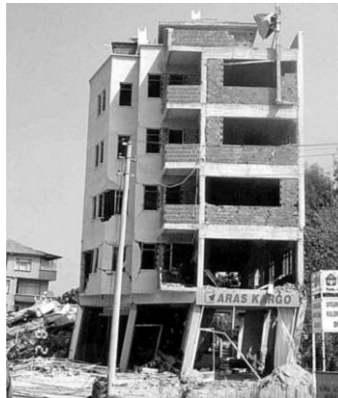
Figure 1 Formulation of soft storey mechanism during Turkey earthquake, 1999 (Sezen, 2003)
