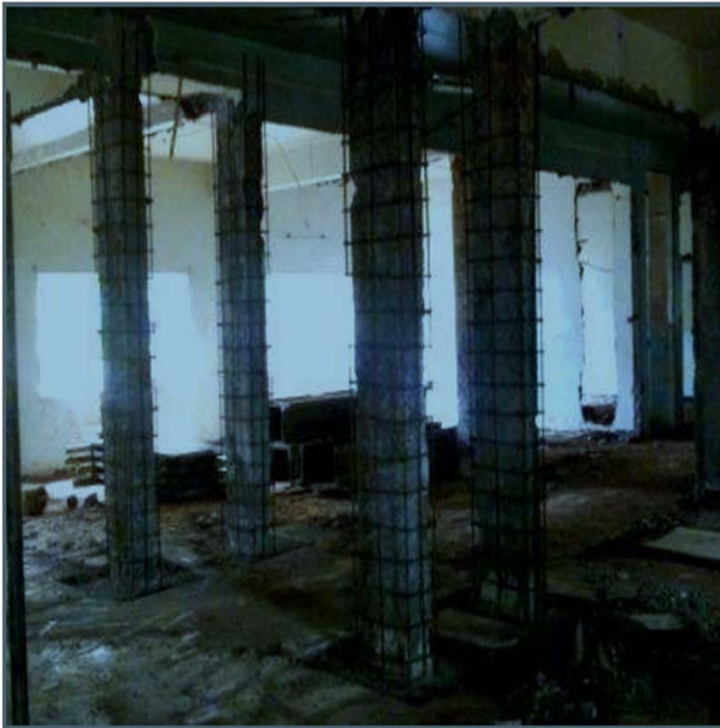
Figure 3 Additional Reinforcement & Micro concreting
